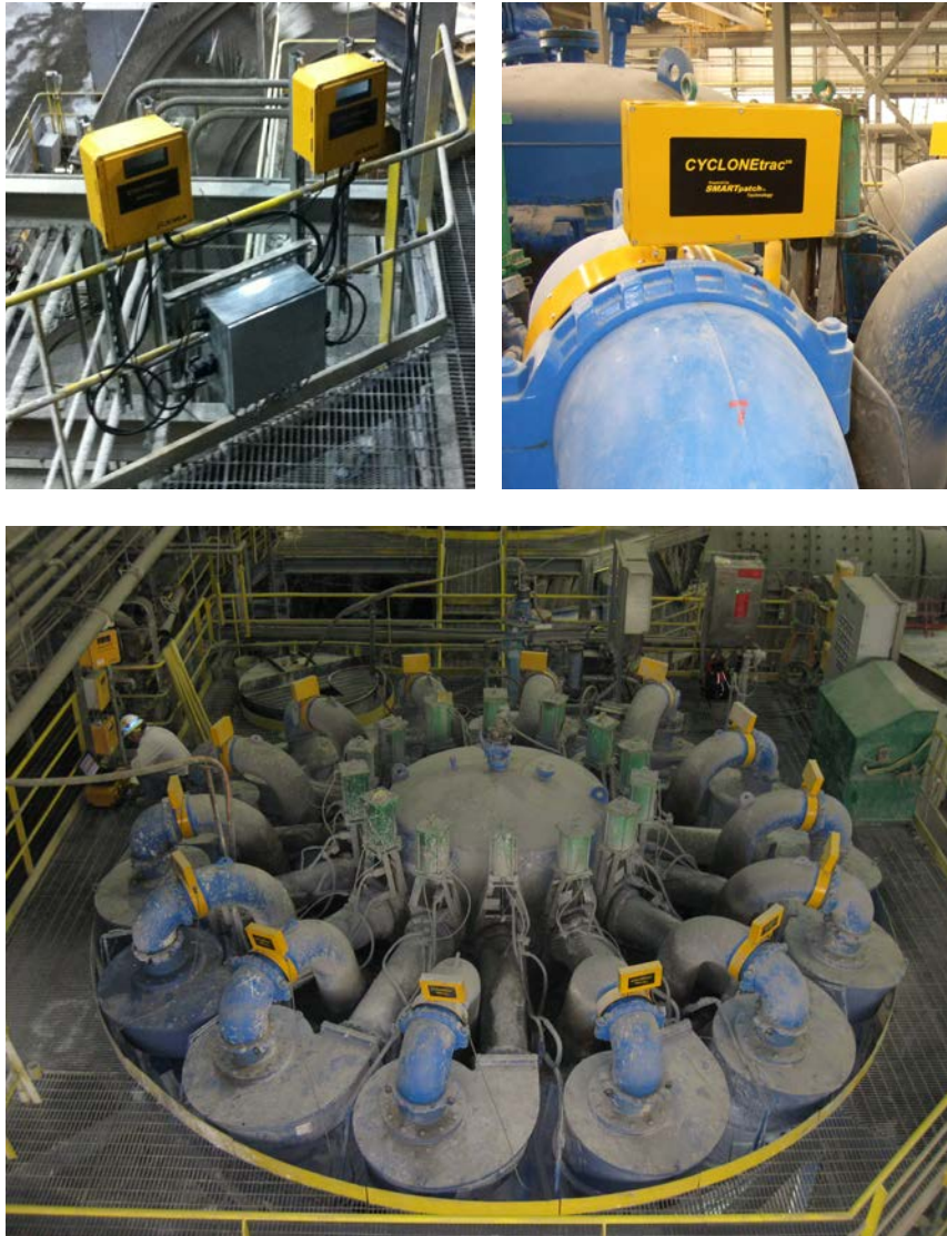
Figure 4 – CYCLONEtrac installed on hydrocyclone battery 8
