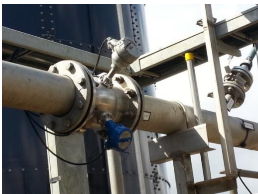
Figure 3: installation in a pipeline
